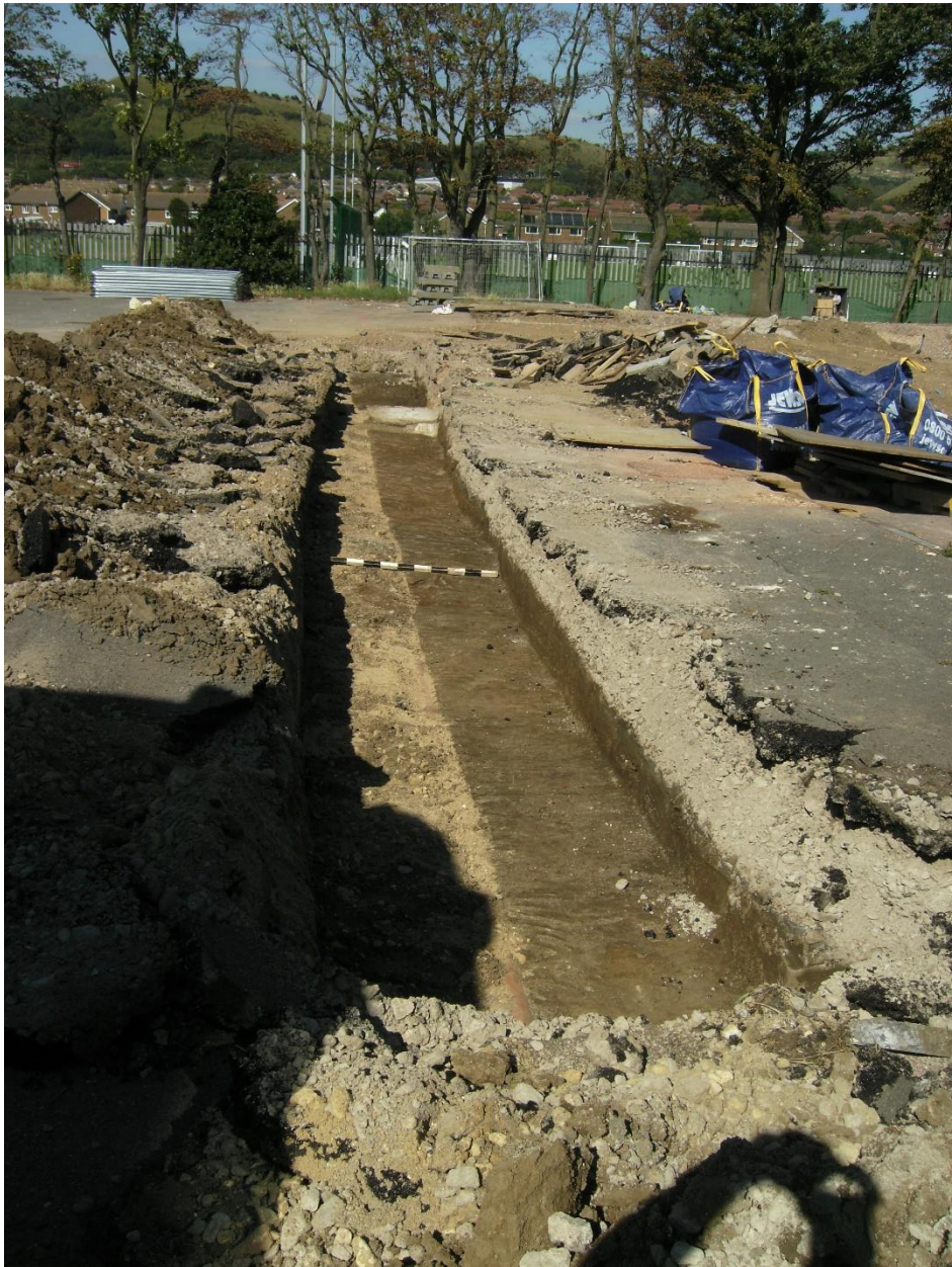
Plate 1. Trench 1 looking north showing the exposed modern service trench on the left (one-metre trench)
